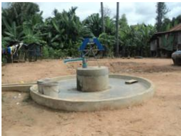
Communal well repair with Rovai pump
