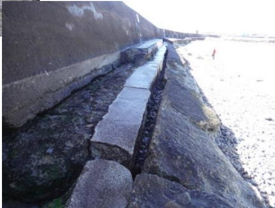
Repair work being undermined
