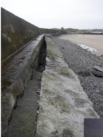
Toe falling away from the wall
