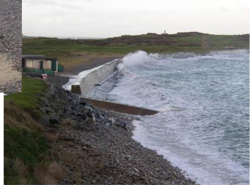
Wave action causing scour
