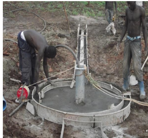
Borehole nearing completion
