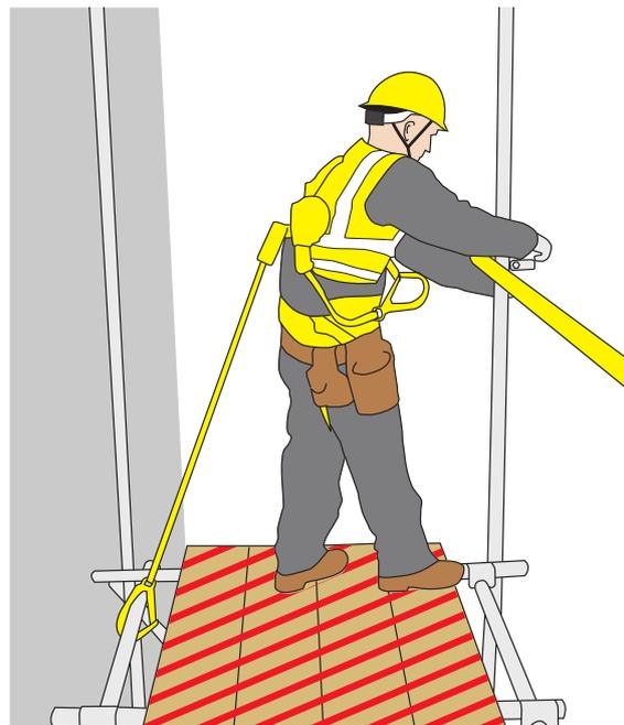
Figure 13: Example of Personal Fall Protection.
