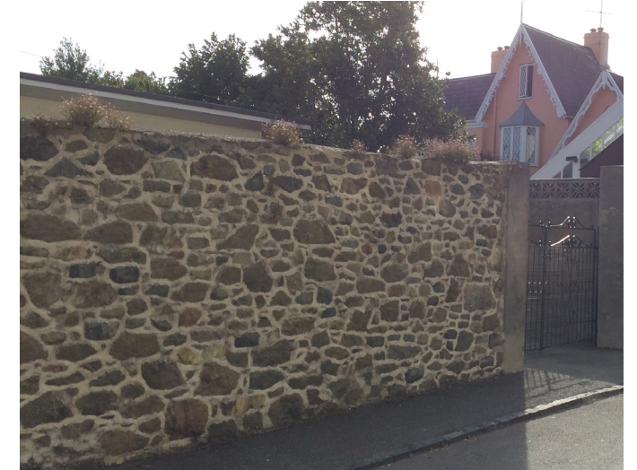
9: Random rubble stonework opposite Housing Allocation site on La Couperderie
