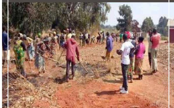
Villagers backfilling trench for pipework
