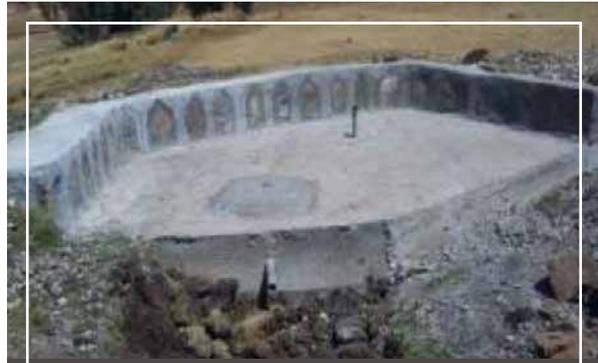
The construction of Sayntew spring. 10m<sup>3</sup> sandwiched Masonry service reservoir
