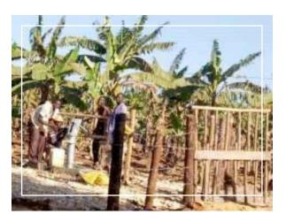
Work on drilling the bore hole, finishing off the concrete base of the pump and showing the new water source in operation and fully protected from animals, etc.
