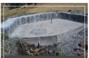
The construction of Sayntew spring. 10m<sup>3</sup> sandwiched Masonry service reservoir
