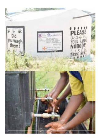
Finally, the report confirmed that, in conjunction with the hygiene training, hand washing stations were set up at each of the schools. These are 1,000-liter plastic tanks fitted with four taps. The health clubs and school management are responsible for making sure tanks are filled with water and that a cleaning agent such as soap or ash is available.
