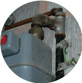
Main bonding connection not made before branch pipework
