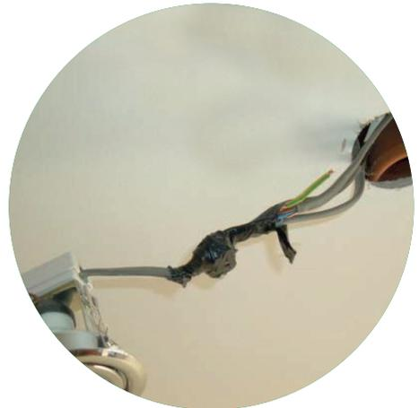
*Unsatisfactory connection to a downlighter, requiring a Code C2*
