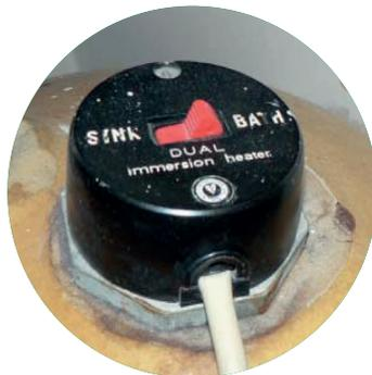
Older immersion heater without thermal cut-out
