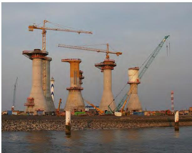
Figure 2.2 Example Concrete Gravity Foundations/Structures – Thornton Bank project
