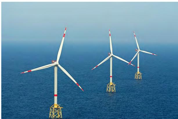
Figure 2.4 Examples of Turbines on a Jacket Structure
