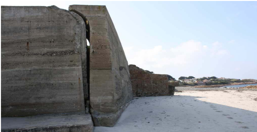
Photo Showing Gap between Bunker and External Facing Wall
