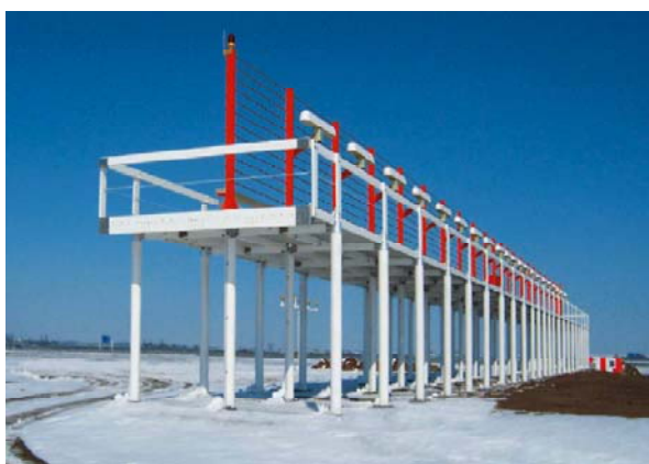
An ILS localiser installation on a 6m high Euro Pole structure.
