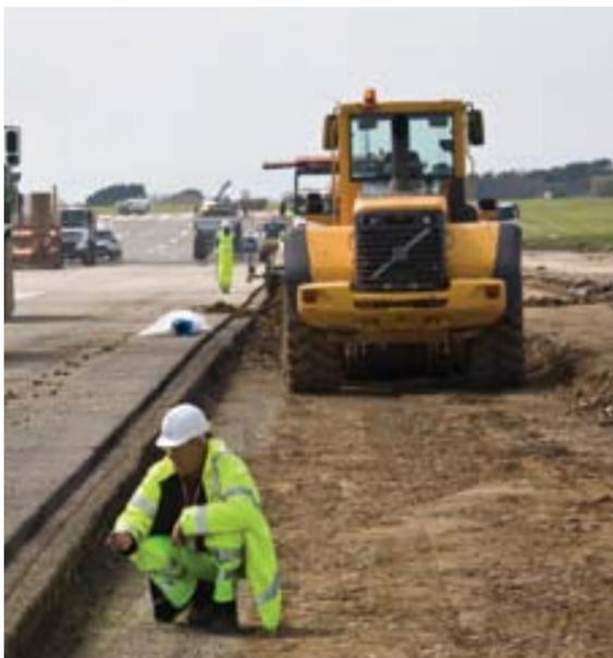
The edges of the runway are being reconstructed prior to the main overlaying operation this summer.
