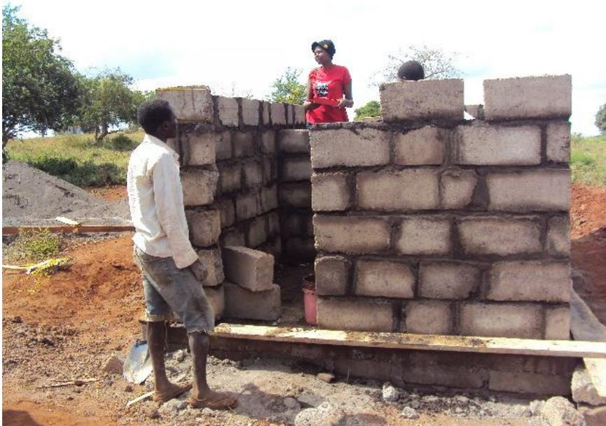
**Figure 5 Toilets and Bathrooms under construction**
