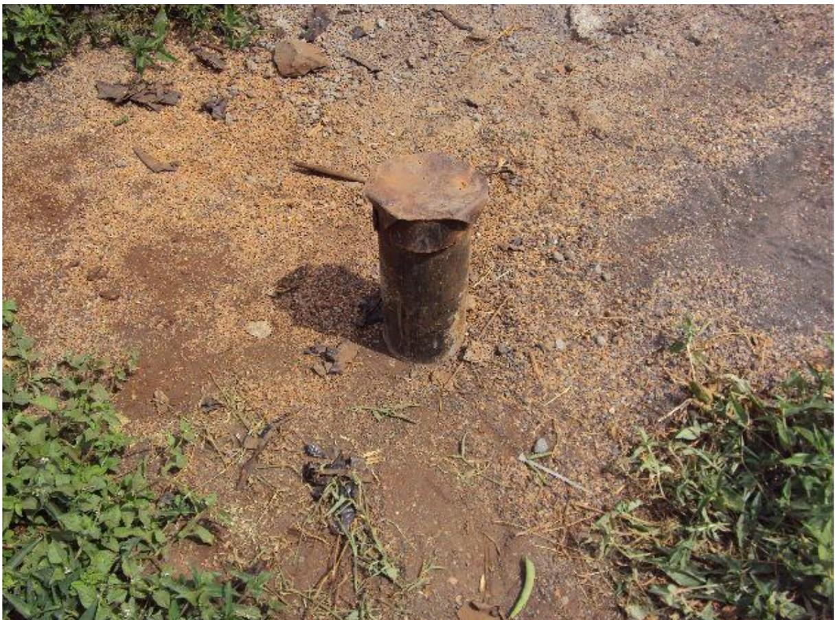
**Figure 1—Drilled borehole cased and ready for equipping**
