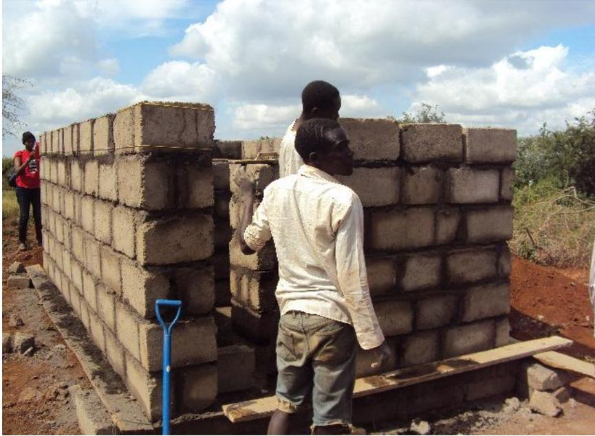
**Figure 4 Sanitation Facilities under Construction (these are part of equipping the borehole to facilitate the communities as they use the boreholes and bring the animals to take water.)**
