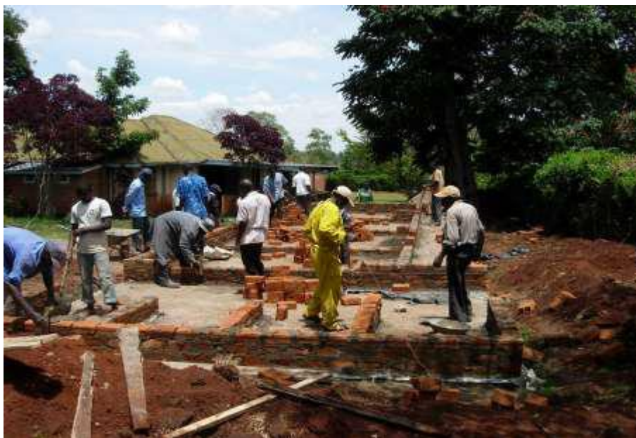
Picture 6 – Construction work on the foundations for the new hospital wards
