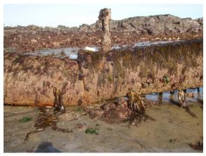
**Short Sea Outfall** – Air Vent Opening along length of outfall pipe – damage caused during February 2014 storm event
