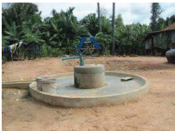
Communal well repair with Rovai pump
