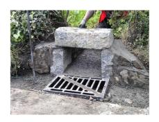
In 2014, a number of special projects were undertaken, especially with regard to surface water drainage. One project included the creation of a new granite servitude at Les Prevosts. Following construction, the granite was topped with earth and turfed to continue the existing line and maintain the rural appearance. This has significantly eased the flooding problems which had been quite serious in this area.
